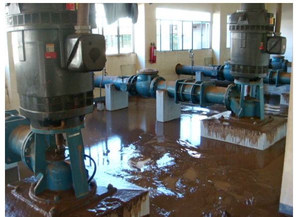
Flooded pumps at COWD's main booster pumping station.
