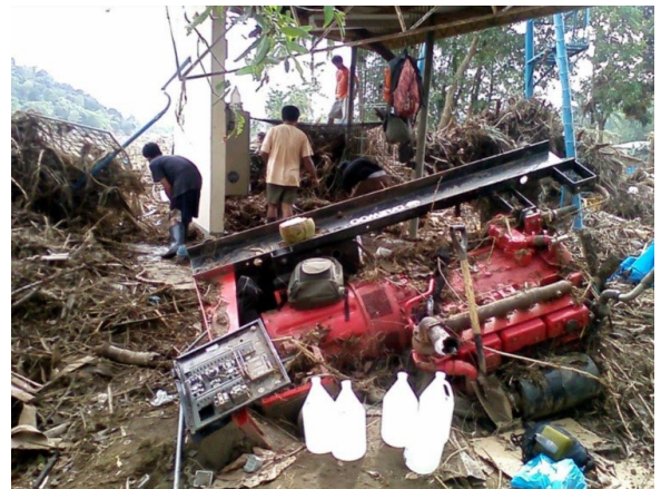
Damaged generator at one of COWD's production wells.
