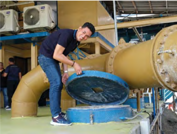
Philippines — Cagayan de Oro City Water District’s operator supervisor Anthony Castro checks the water level of the collector well at Macasandig booster station. The collector well is now completely sealed to allow it to remain in operation, even in case of flooding of the booster station by the Cagayan de Oro river.
