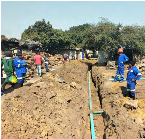
Uganda – Constructing a water distribution system. ▾
