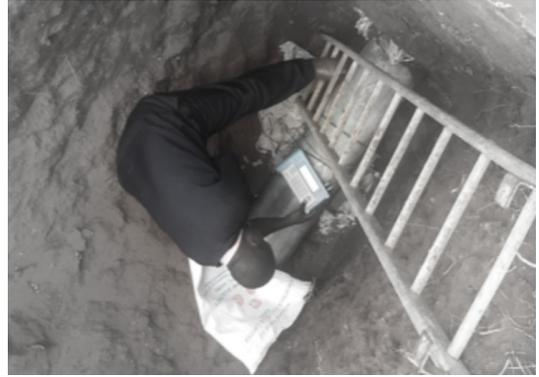
*NRW Technician doing Flow measurement using the UFM*
