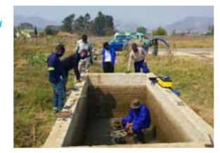
Zimbabwe – Local knowledge exchange from a plumber in Harare explaining to the technical team in Mutare how to set and maintain a pressure reduction valve. This will reduce the high occurring pressures in the mountainous area of Mutare.
